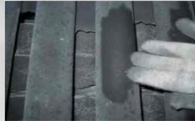
After side pipe
