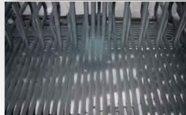
After ceiling pipe
